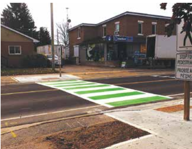
A green and white safety crosswalk was recently installed in the heart of Lafontaine.
